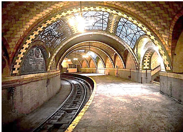
Front endpapers, City Hall Station
