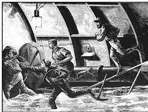
‘sandhogs’ running to escape a leak in the airlock of an underwater tunnel
