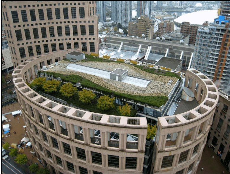
Vancouver Public Library, showing circular design as well as the 'green' roof top garden
